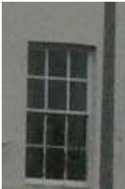
Green Hall Showing Six-over-Six Sashes without Horns
