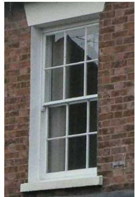
Late Nineteenth Century Building Showing Six-over-Six Sashes with Horns
