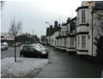
Triangular Site at North End of Lichfield Road
