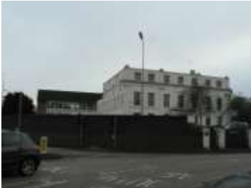
Late Twentieth Century Extension to Rear of Green Hall
