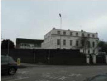
1980s extension visible to rear of Green Hall
